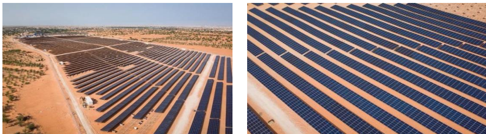
Figure 1. Aerial views of the 50MWp plant, © CLEMESY
