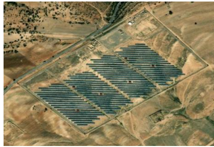
Figure 1. Sidi Bel-Abbes photovoltaic power plant
