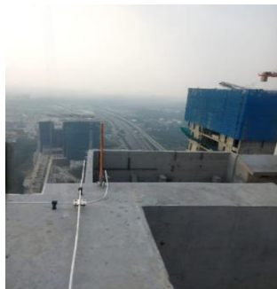
Figure 4. Installation of a vertical air terminal
