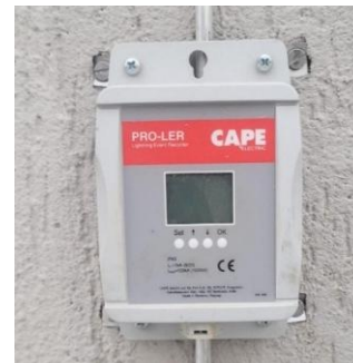
Figure 5. Installation of the lightning event counter
