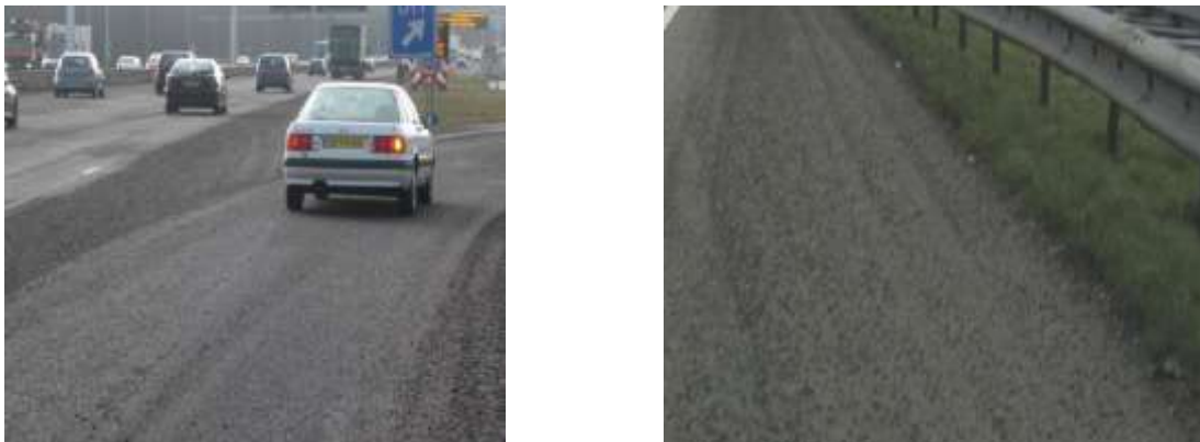
Figure 2. Serious ravelling on highways Amsterdam A1 (left) and The Hague A4 (right)
