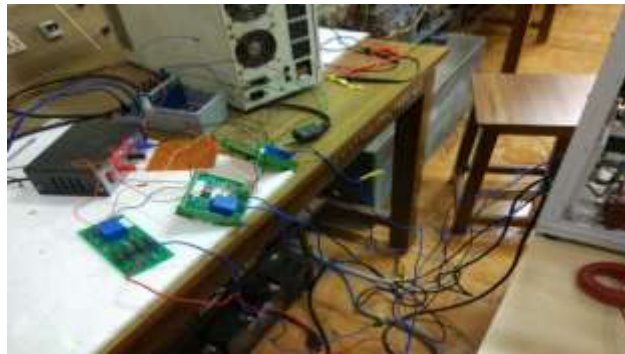
Figure 2. Power quality monitoring system implemented
